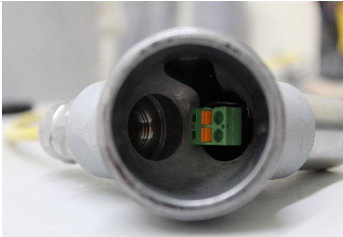
Figure 4 – Typical Inspection Photo
