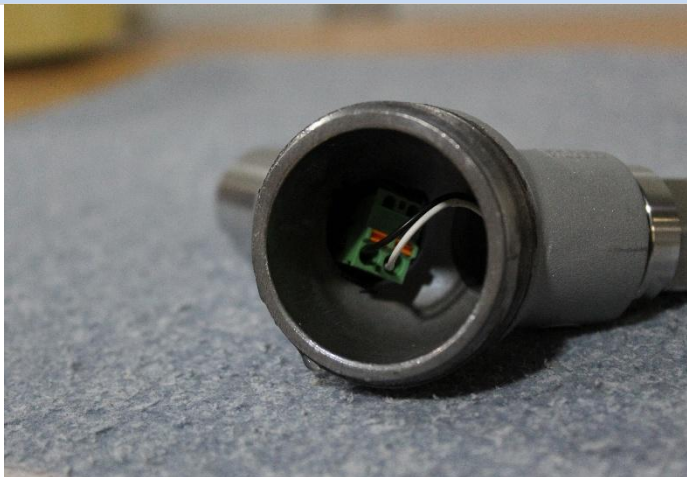
Figure 12 – Typical Inspection Photo
